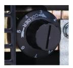
Knob-type mechanical thermostat for selection of set point temperature is located in the toe grille below the door
